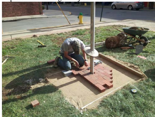
Above: John Buckles laying brick around the flagpole.
